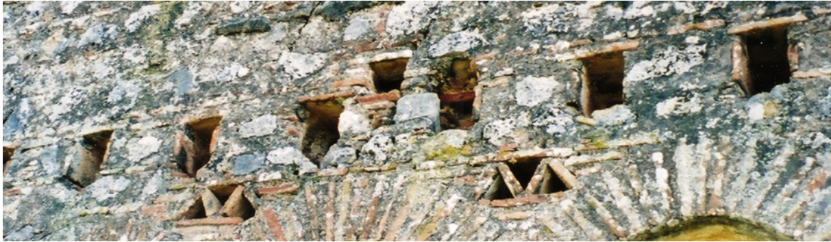
Fig. 52. Mastro, Ag. Ioannis Riganas / Episkopi. Detail of the W façade.
